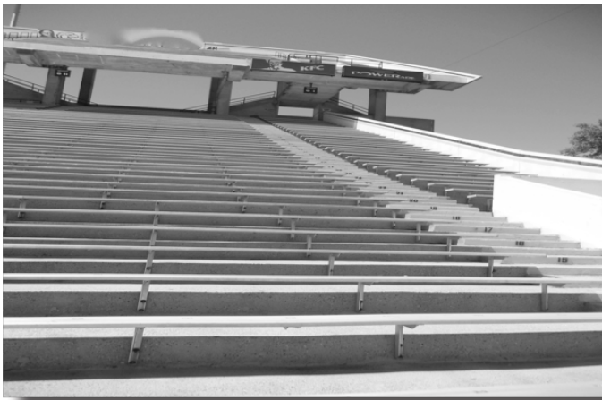
Figure 2. Stair height of bleachers is regulated to accommodate persons with mobility.
