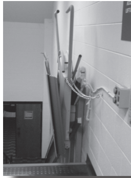
Figure 8. Lifts assist those who are unable to ascend stairways.
