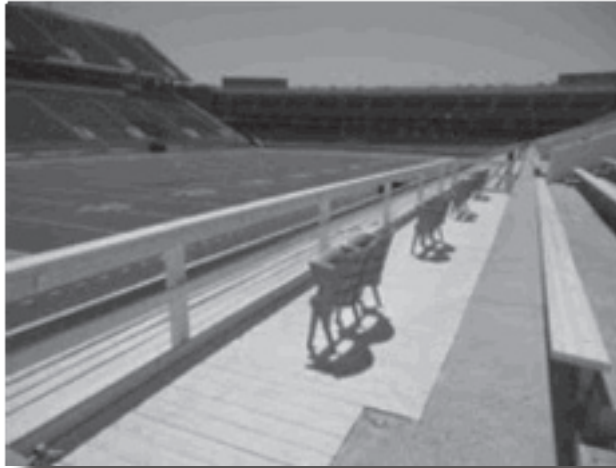
Figure 3. The number of wheelchair accessible seats falls short of current ADA guidelines.
